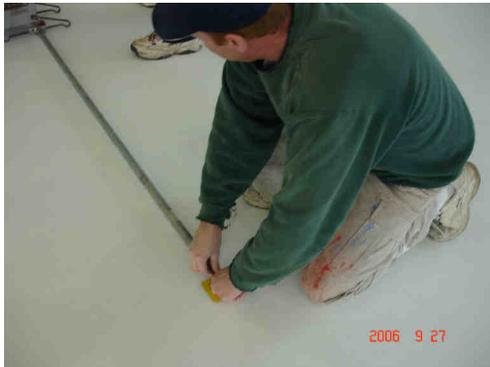
For curling circles, a bolt is frozen into the center of the circle (house) during installation of first layer of new arena ice. A small metal plate with raised hollow center fits over the bolt.
